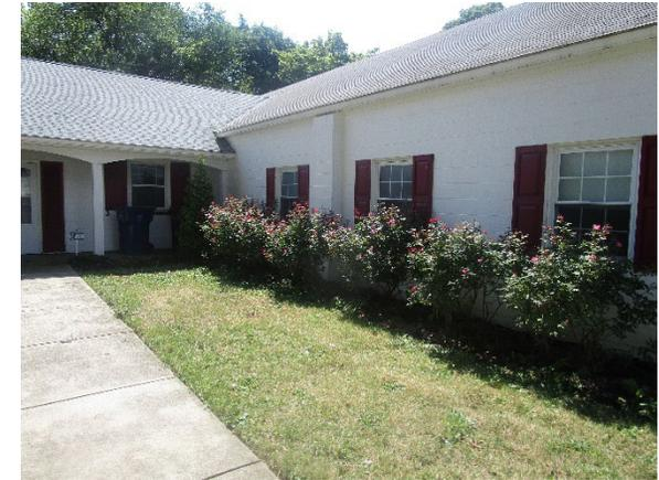
A rain garden can be installed at the northwest corner of the building to capture, treat, and infiltrate the stormwater runoff from the rooftop. Two downspouts on the north side of the building can be led to the rain garden. A preliminary soil assessment suggests that more soil testing would be required before determining the soil's suitability for green infrastructure.
