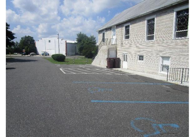
A rain garden can be installed on the east side of the building to capture, treat, and infiltrate the stormwater from the rooftop. Parking spaces on the west side of the building can be replaced with pervious pavement. A preliminary soil assessment suggests that more soil testing would be required before determining the soil's suitability for green infrastructure.
